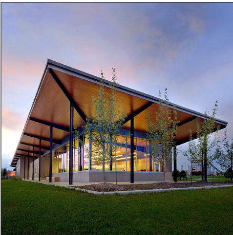
© Gayle Babcock, Architectural Imageworks L.L.C.
