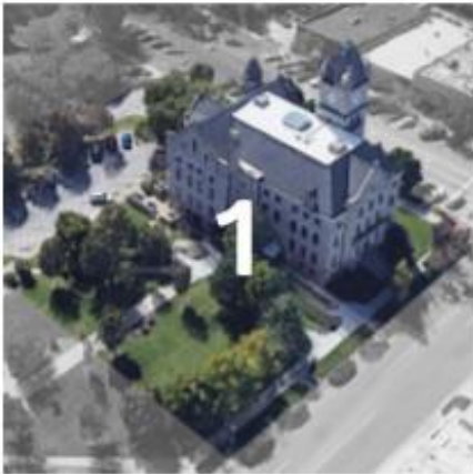
Historic Courthouse Renovation
