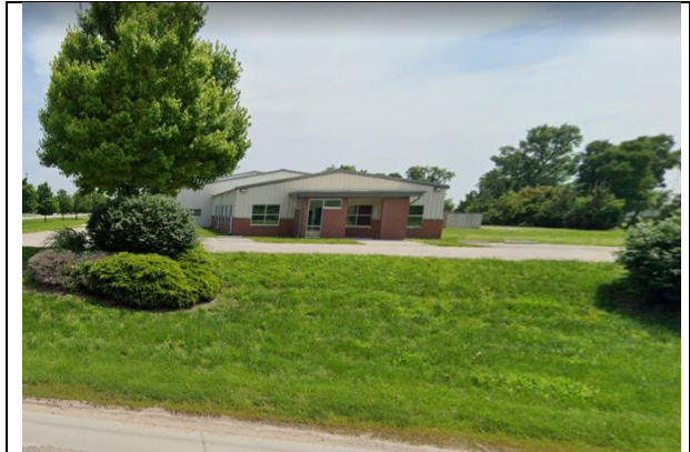
Figure 3a. View from Hwy 24/59 / E. 1450 Road
