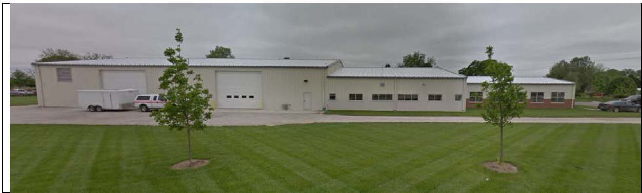
Figure 3b. View from N 1823 Road
