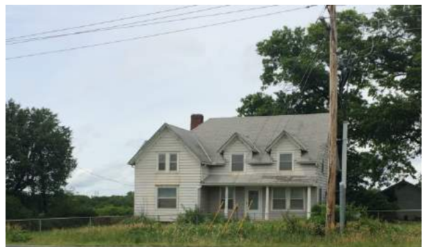
High amperage power line on Farmer's Turnpike
