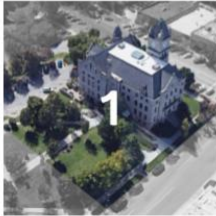
Historic Courthouse Renovation
