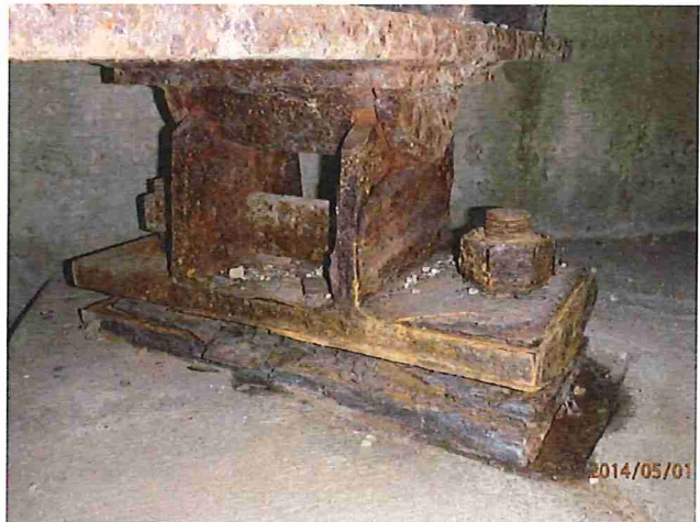
Existing steel bearing
