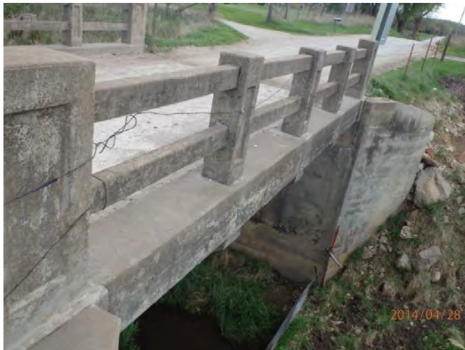
Bridge prior to replacement
