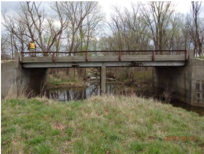
Existing bridge in 2016
