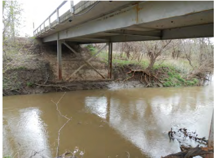
Existing steel girders
