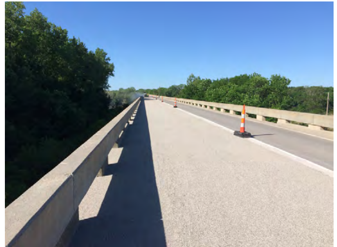
Overlay Route 1029 Kansas River Bridge completed 2017
