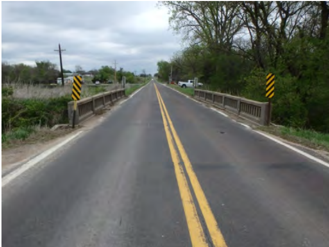
Roadway before replacement
