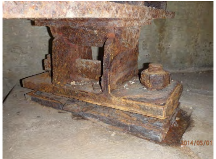
Existing steel bearing
