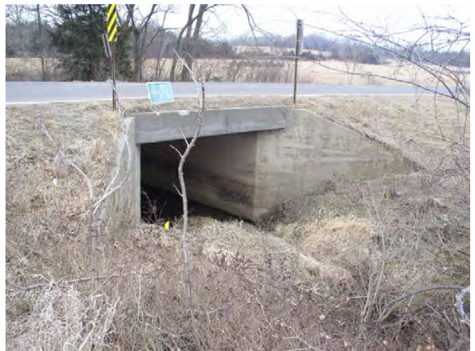
Existing narrow culvert
