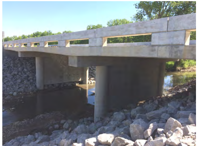
Replacement completed May 2017
