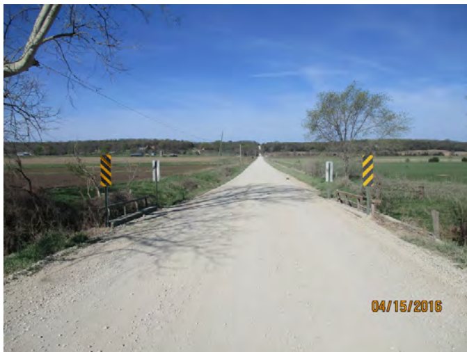
Existing narrow culvert
