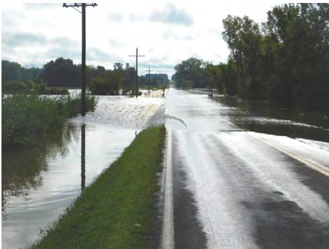
N 1000 RD flooded July 2017
