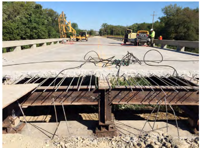
Repair work on bridge 1186-1500
