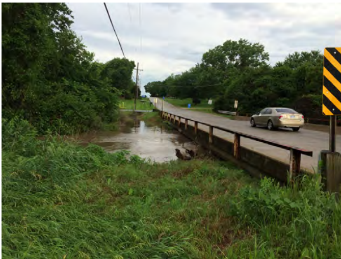
High flow at bridge 1100-1330
