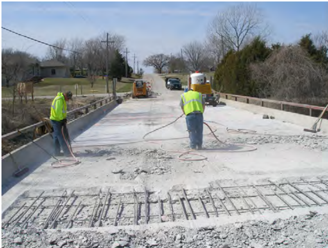
Concrete deck repairs
