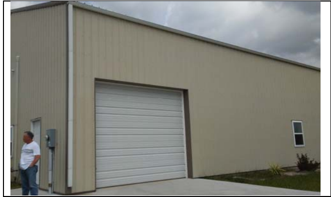
Figure 6 Existing warehouse building.
