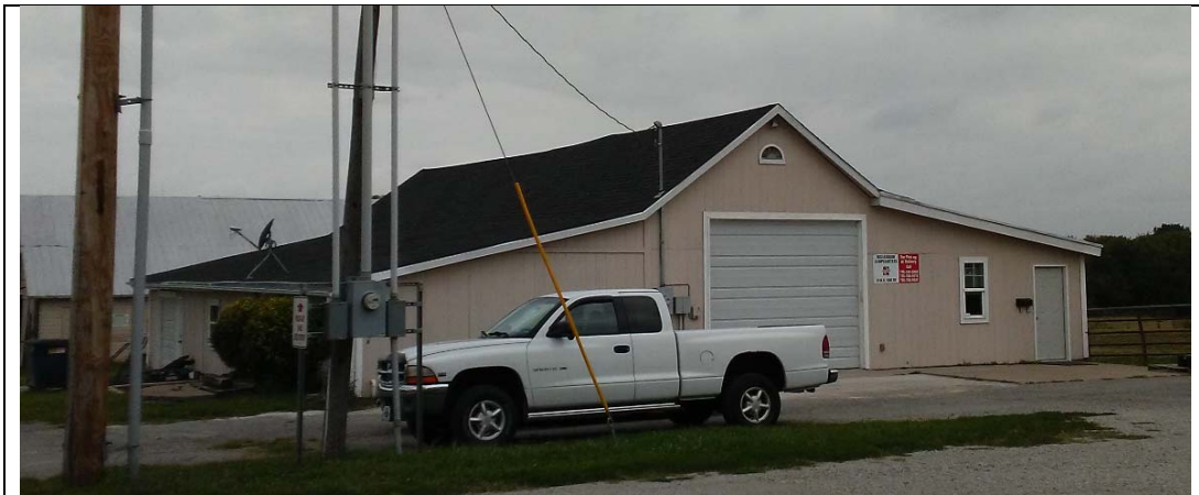
Figure 7. Converted barn used for production area, and storage of product.
