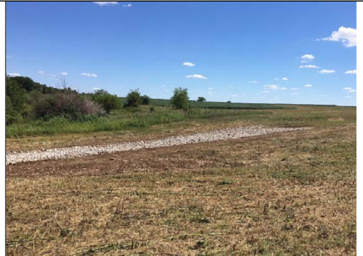
Figure 1. Rock placed along spillway.
