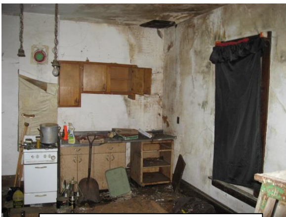
Kitchen Before Rehabilitation
