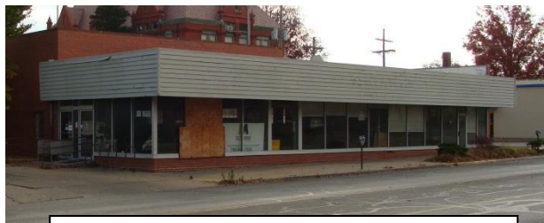
1040 Vermont Street Before Renovation
