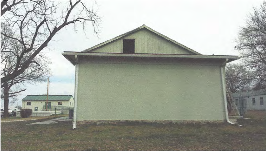
Means Home - West façade with attic access door open for inspection.
