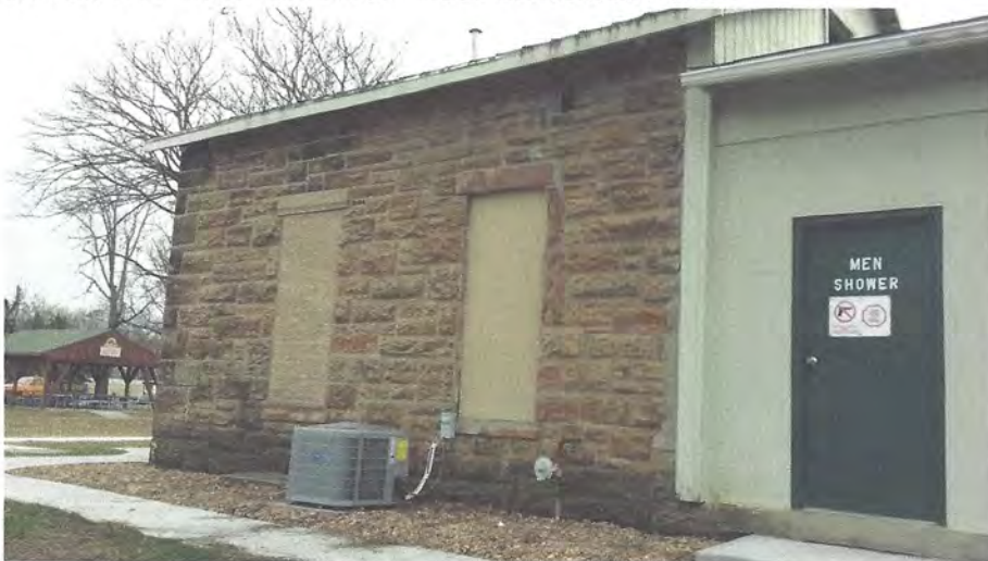
The South Façade showing location of “Kitchen Door” near an outside well.
