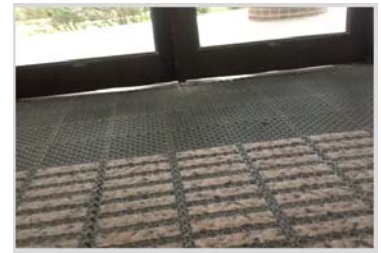
Visible Gap Under Exterior Doors at The Sports Pavilion
