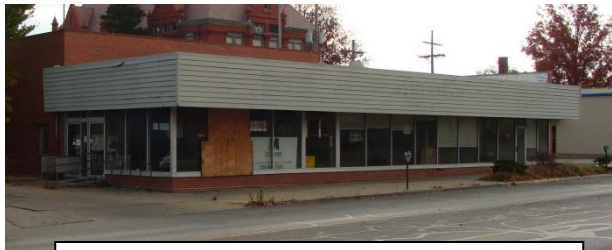
1040 Vermont Street Before Renovation
