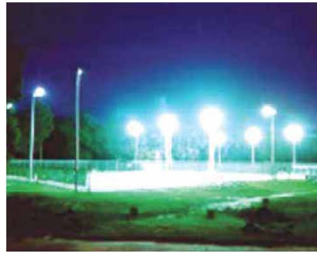
Floodlighting produces uncontrolled light.
