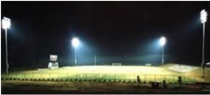
Figure 3. Example of reduced glare from shielded sports lighting.
