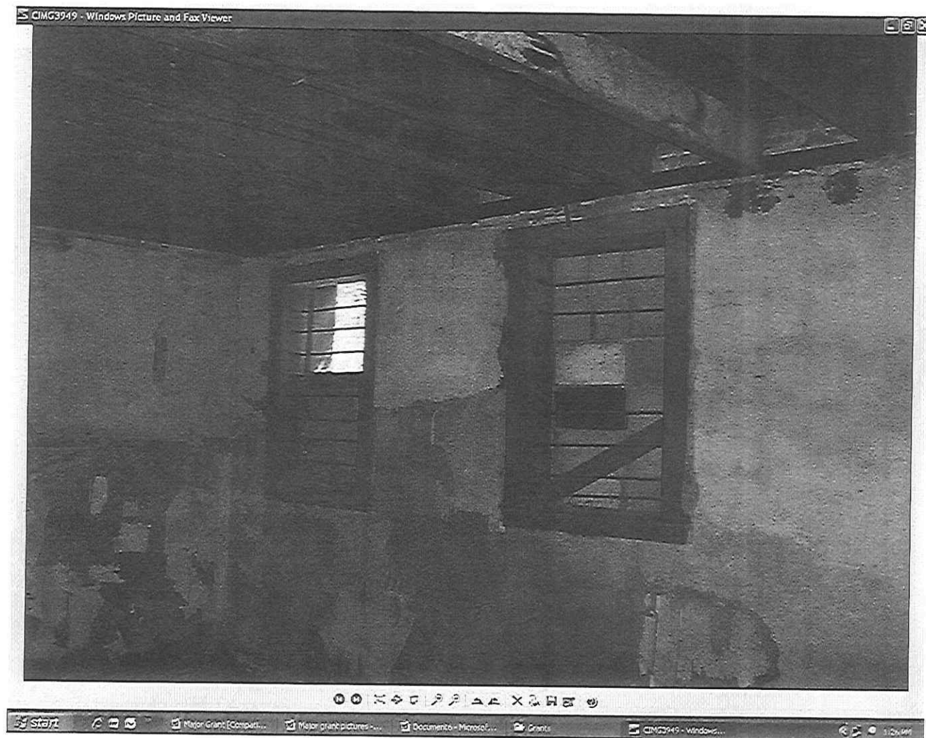
Interior of 720 Main, second room, first floor, south wall.
