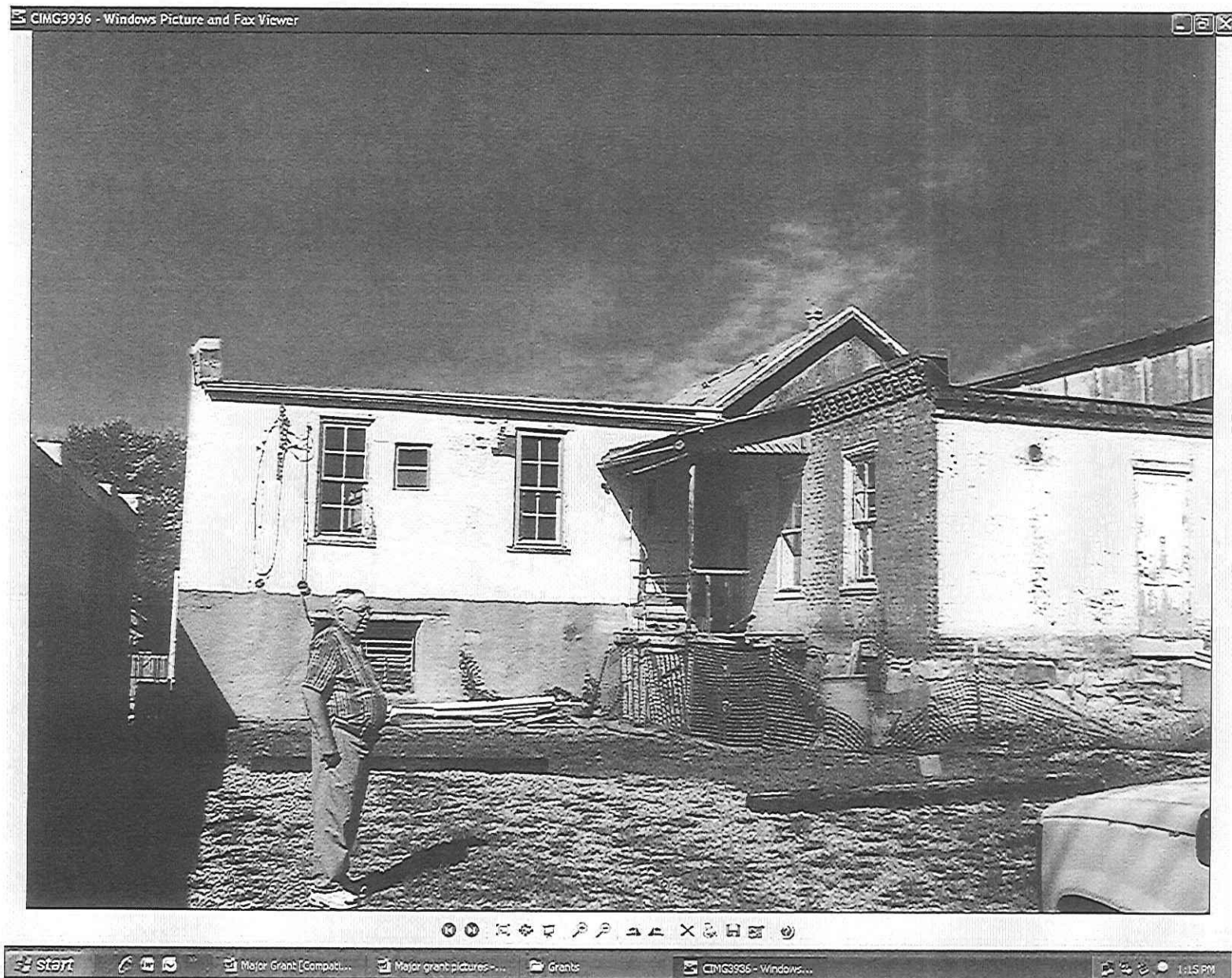
View of 720 and 722 from the rear, looking Northwest.
