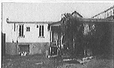
Caption: Douglas Co., Eudora, 720 MAIN ST., 09/08/2009, rear, photo taken by Cindy Higgins
