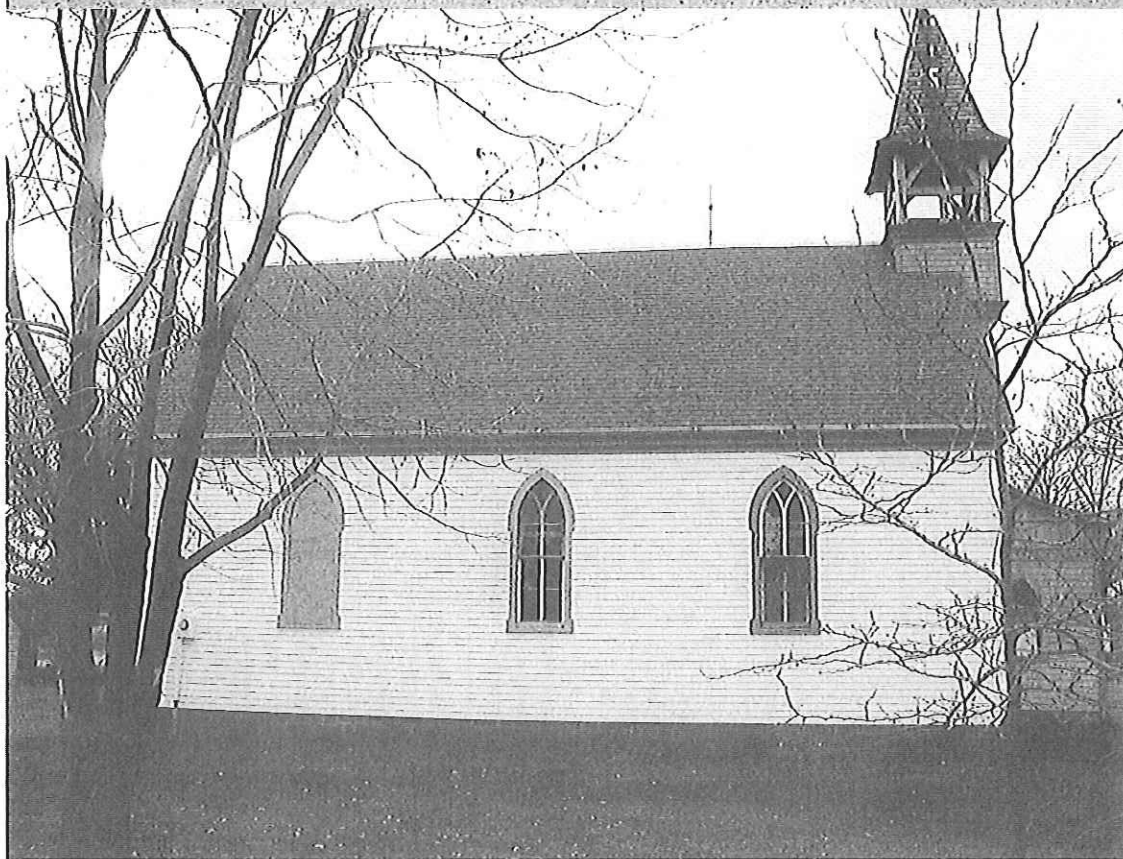
Sanctuary, North side, before and after Preservation Phase I work, 2004-2006
