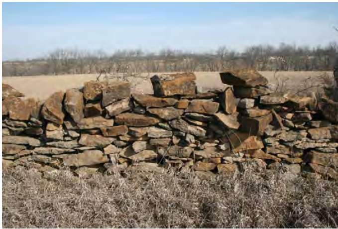
Stone Fence – 1581 E 400 Rd
