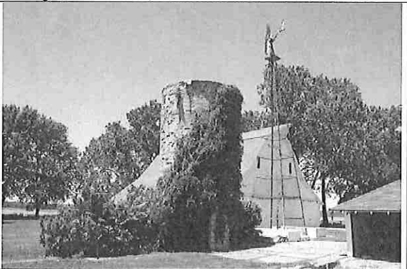
Water Tank & Windmill – 1359 N 1900 Rd
