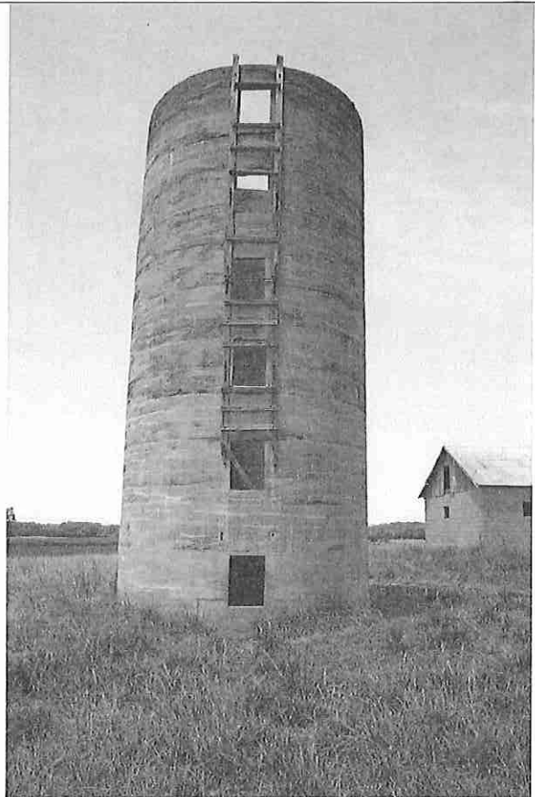
Adam Schick Concrete Silo – 677 E 1700 Rd
