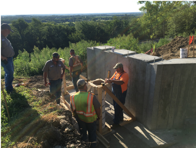
Foundation construction by Public Works crews
