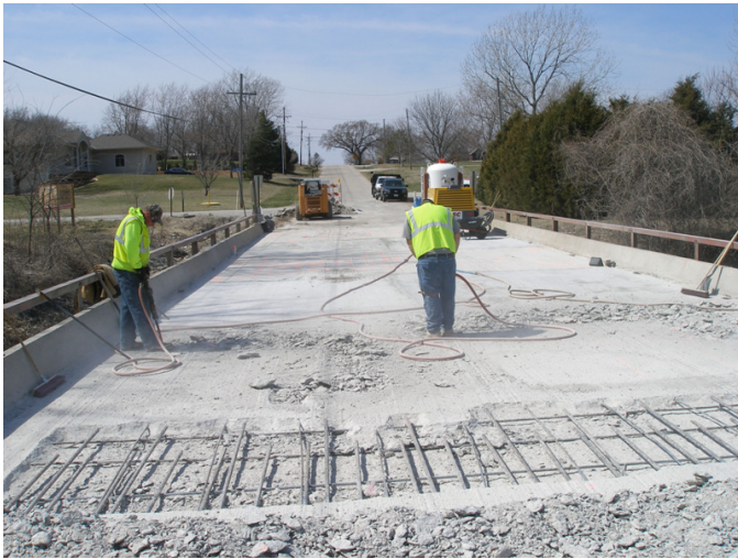
Concrete deck repairs
