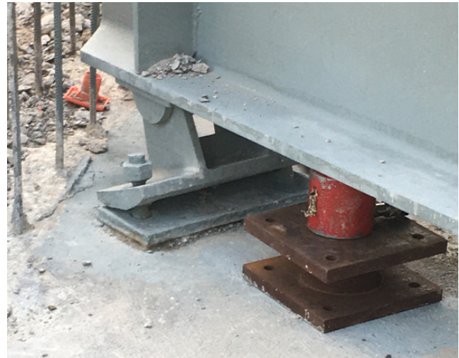
Replacement bearing installation
