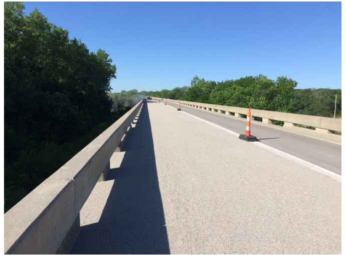
Overlay Route 1029 Kansas River Bridge completed 2017
