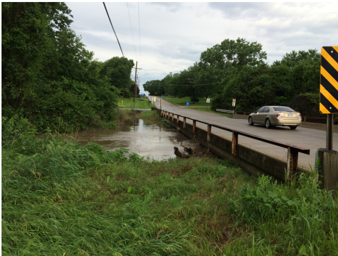
High flow at bridge 1100-1330
