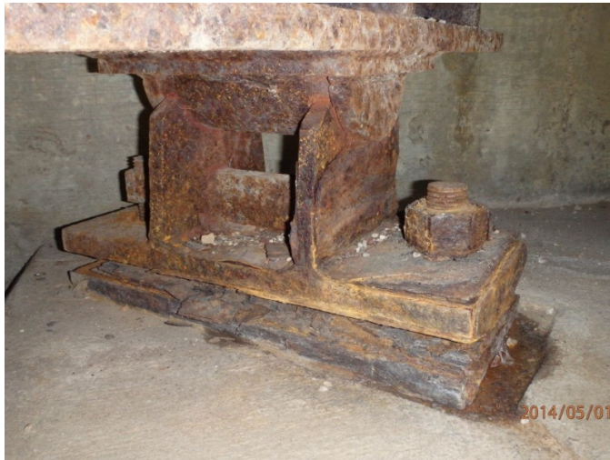
Existing steel rocker bearing
