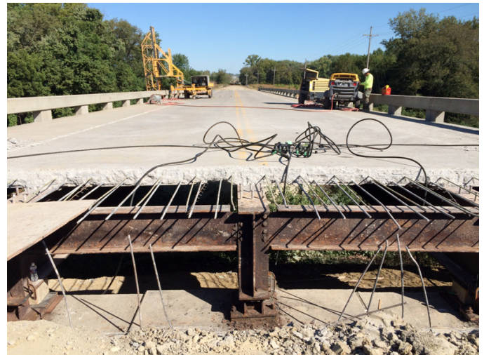
Repair work on bridge 1186-1500
