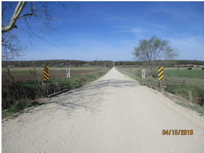
Existing narrow culvert
