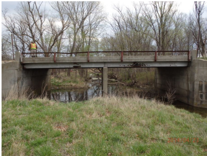
Existing bridge in 2016
