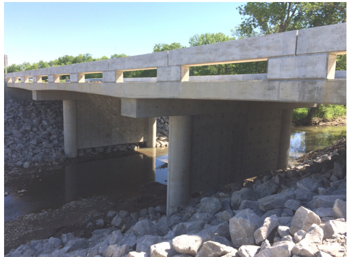
Replacement completed May 2017
