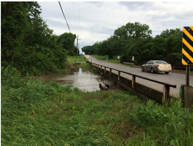
High flow at bridge 1100-1330
