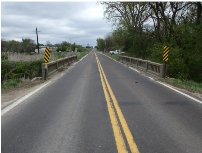
Roadway before replacement
