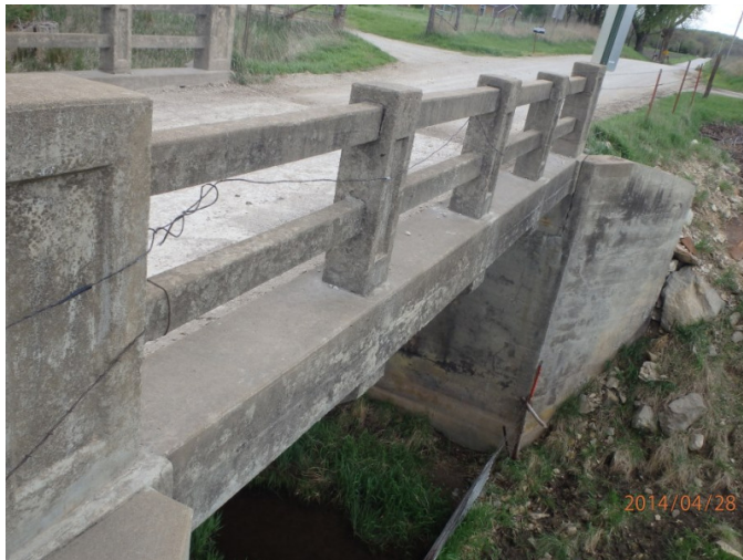
Bridge prior to replacement
