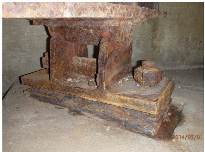
Existing steel bearing
