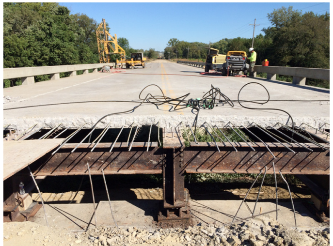
Repair work on bridge 1186-1500
