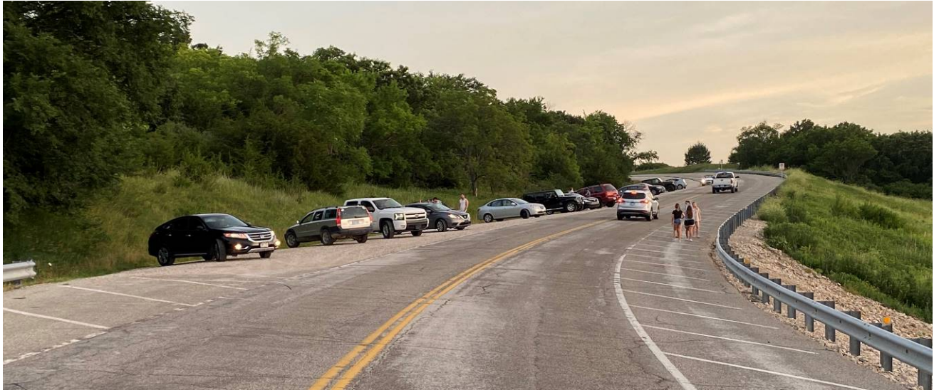
South end of the dam road looking south
