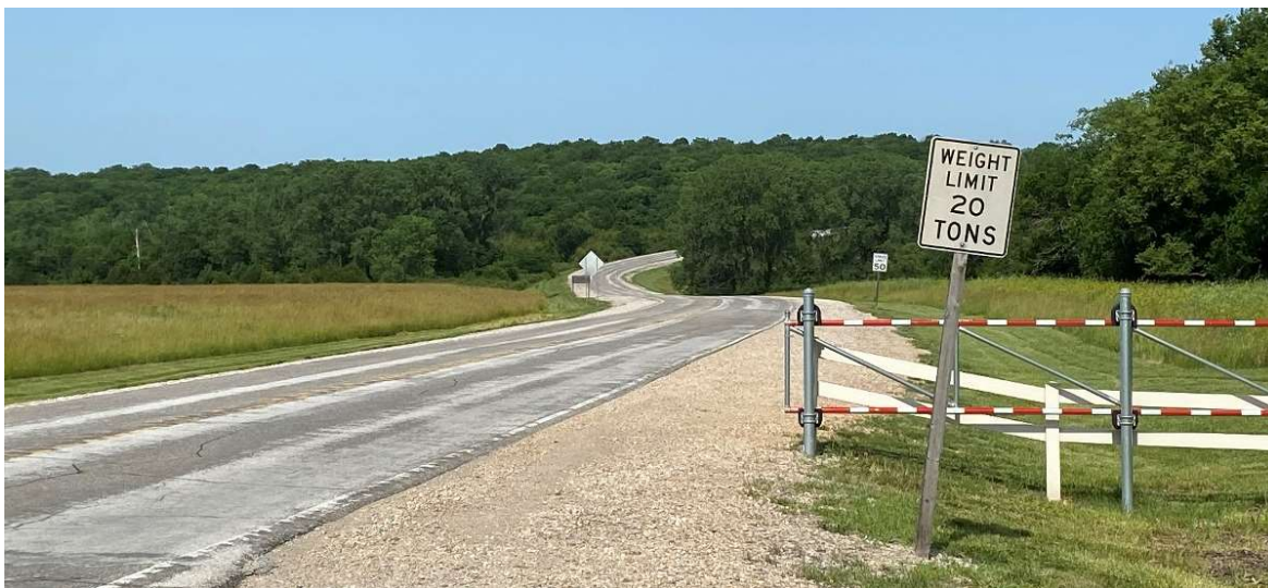
N1150 Road “Dam Road” looking west
