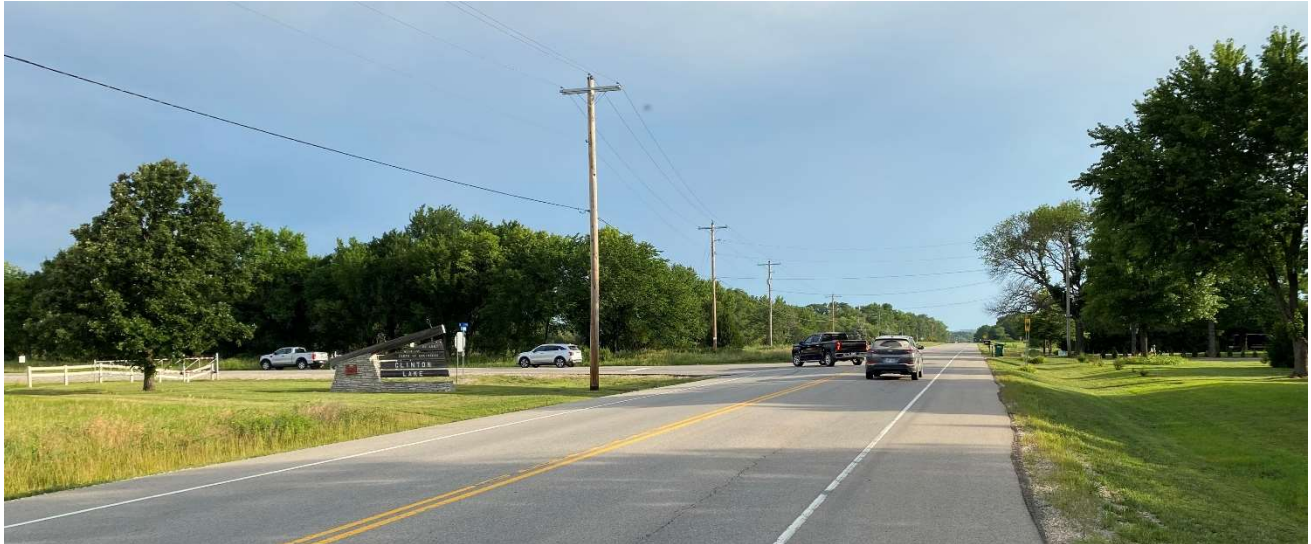
E1000 Road northbound traffic diverting over Clinton Dam
