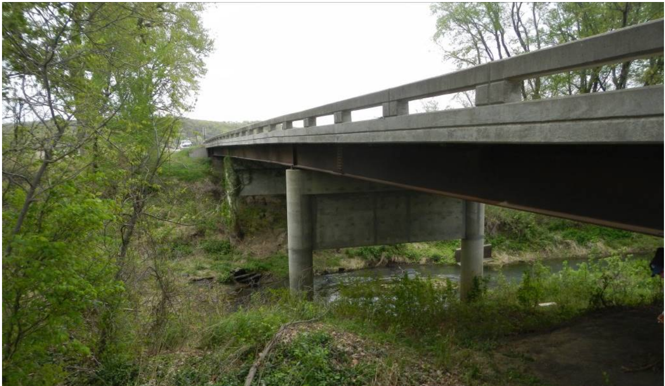
Existing Wakarusa River Bridge at E1150 Road
