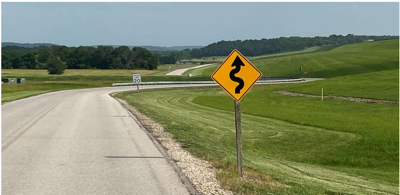
Lower dam road looking south
