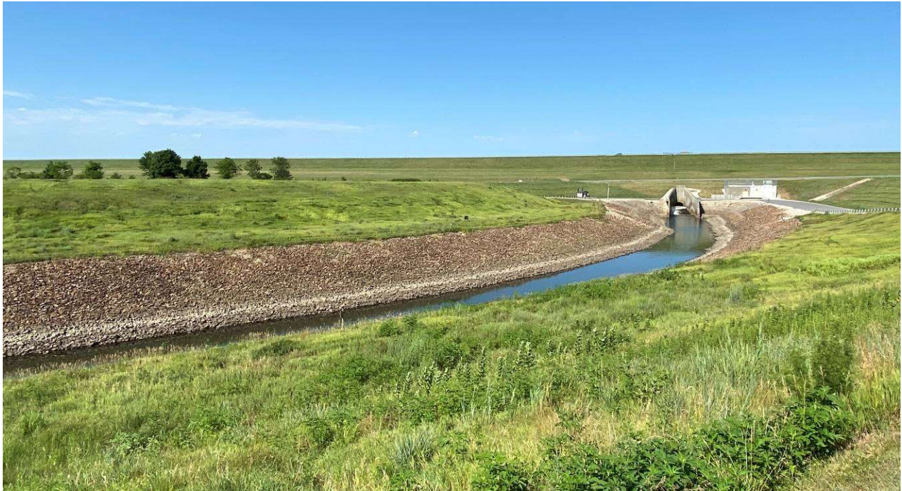
Wakarusa River at the downstream face of Clinton Dam
