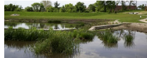
Detention Basins & Constructed Wetlands
