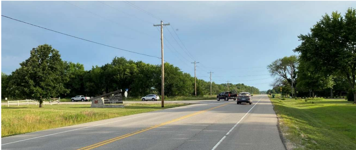
E1000 Road northbound traffic diverting over Clinton Dam
