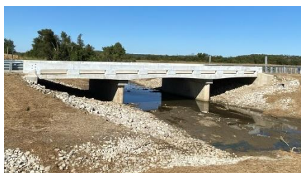
(1) Reinf. Concrete Slab Haunch
