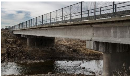
(2) Prestressed Concrete Beam
