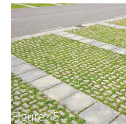
2. Resilient Structure/Permeable Paving
