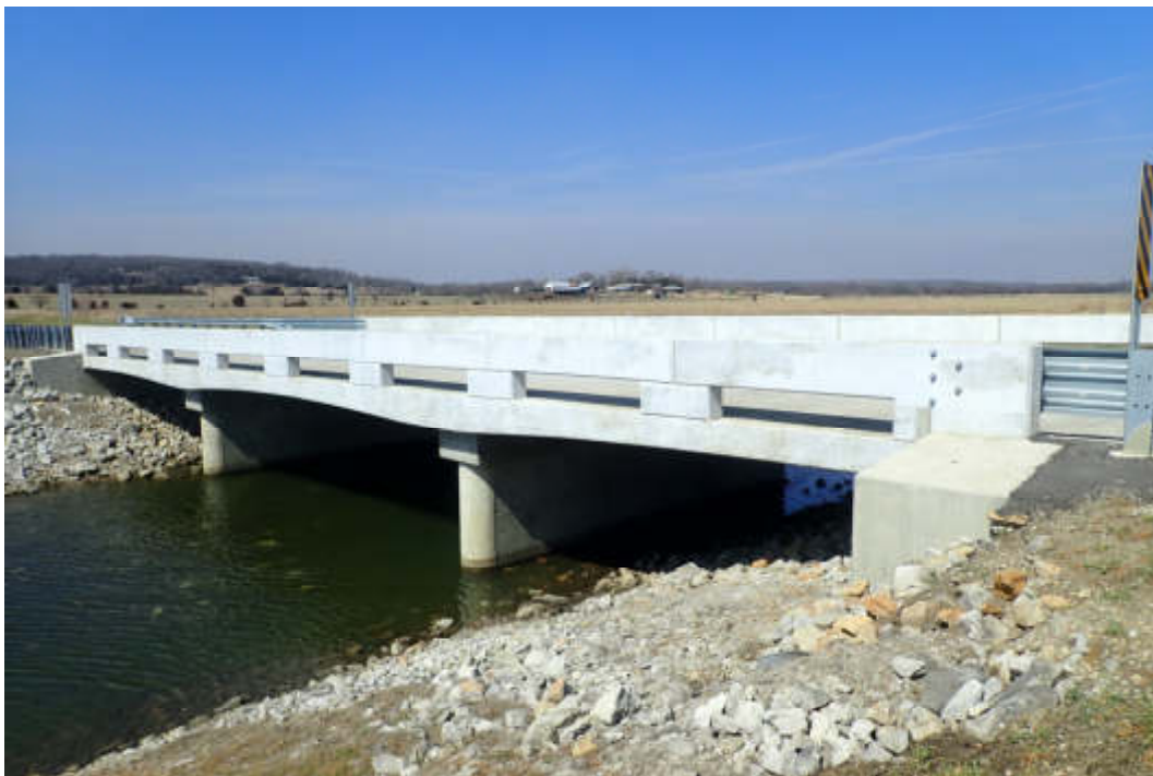
Bridge 0900-1043 constructed in 2021
