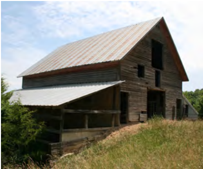
Oakes Barn in Palmyra Township.
