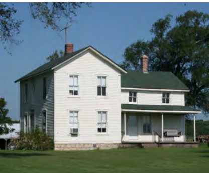
National Folk house from Clinton Township Survey.
