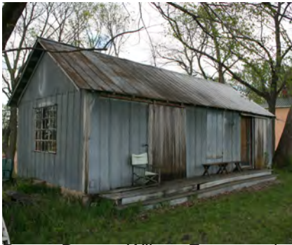
Potato Barn at Wilson Farmstead in Grant Township.
