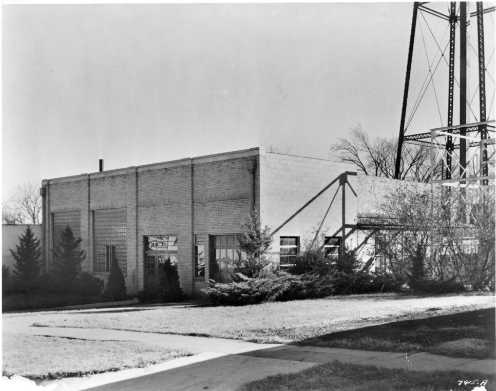
Baldwin City Municipal Electric Plant circa 1945, accessed through Baldwin City Public Works
