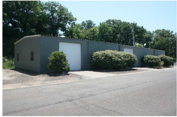
Maintenance Building – 1966 est.
