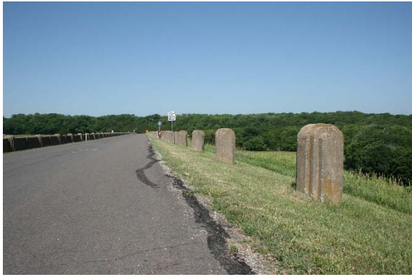
Concrete Pylons – North Side of Dam
