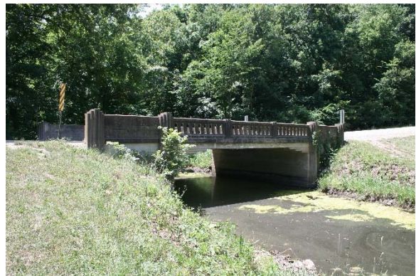
Lone Star Park Bridge No. 2
