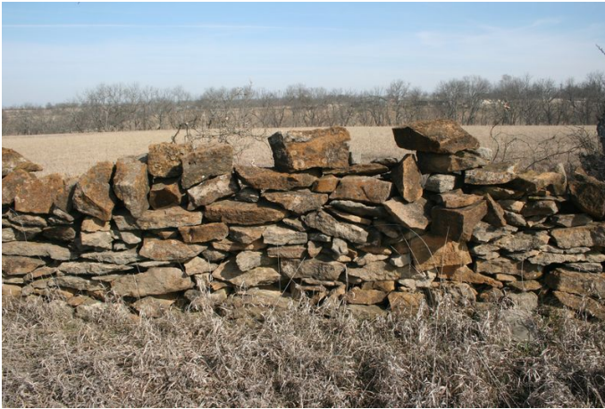
Stone Fence – 1581 E 400 Rd
