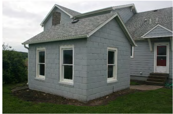
Electric Generating Building
