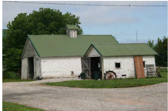
Thome Garage and Granary
